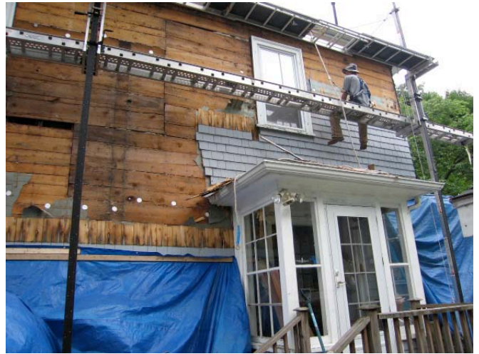
Figure 2. The wall cavities were first dense-packed from the outside with blown cellulose insulation (left). Then the crew stripped off the old cedar shingle siding, focusing on one side of the house at a time to make it easier to protect the house and insulation from the weather (right).
