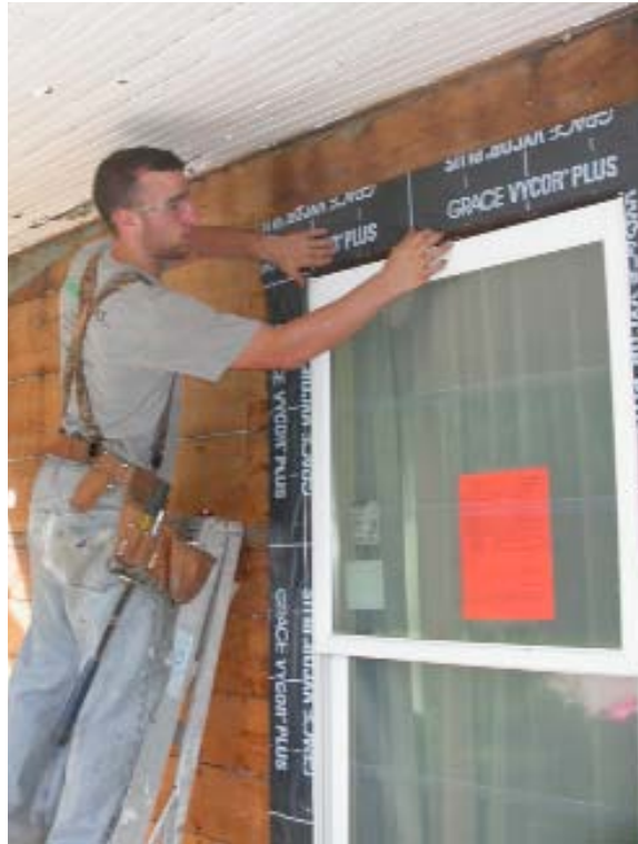
Figure 3. After removing trim from the old windows (this frame was fitted with new jamb liners and replacement sash), crew members filled voids and gaps around the frames with spray foam (A), then taped the frames to the sheathing with self-adhering flashing tape (B). New cedar sill extensions were applied to the sills (C), while the frames were fitted with new 1 3 / 8 -inch-wide Azek jamb extensions (D).
